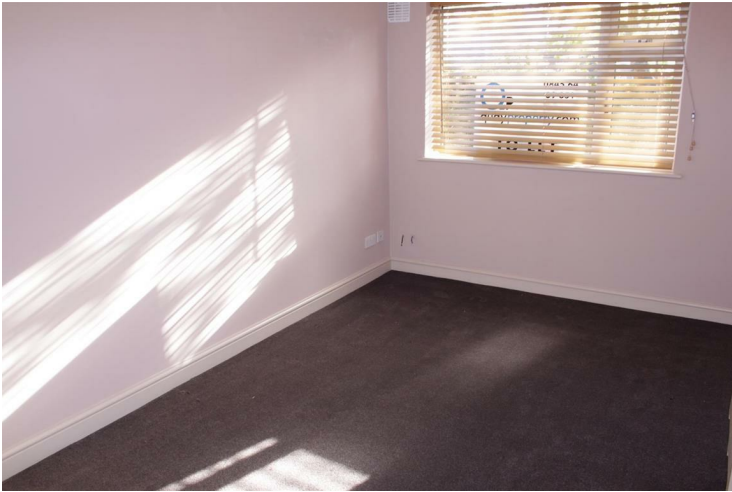
Window to front aspect, Carpeted floor, Power points & Radiator.
